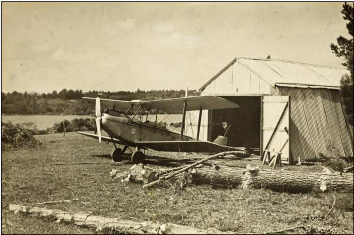
The temporary hangar built by Douglas Mill at Hobsonville
